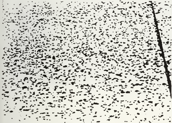
Fig. 3.2.1.1 — Polished pavement
